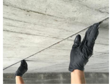
Placing RenewWrap CF carbon fiber bars in slots
