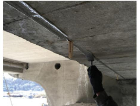
Tooling surface of epoxy
