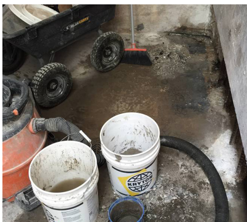
Krystol Plug and Krystol Repair Grout stopped the leaks and repaired the cracks in various areas of the foundation slab and walls.
