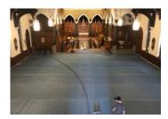
Schönox Renotex® 3D, a multi-dimensional fiber reinforcement fabric, was rolled in place throughout the project area, acting as a decoupling layer between the self-leveling material to come and the poly sheeting on the wood subfloor.
