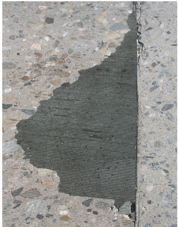
Figure 1: FastPatch DPR after grinding.
